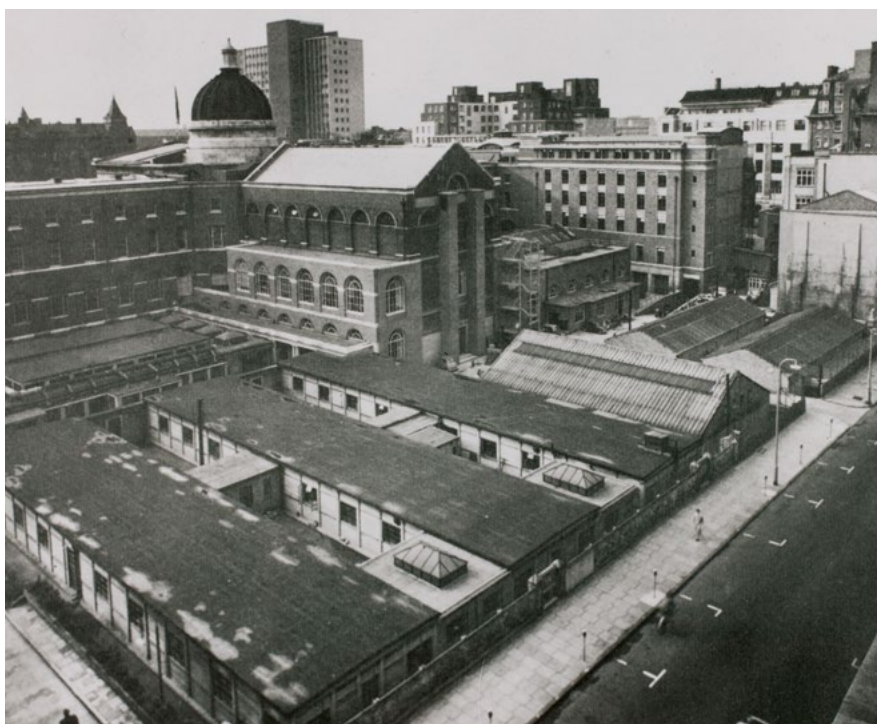
A view of the UCL site from Gordon Street, including many of the post-war huts, that were home to many Students' Union activities. The Student Centre now sits on this site. UCL Special Collections.
