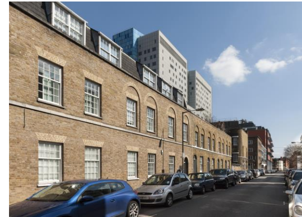
Yvonne Carter Building, Ashfield Street.
