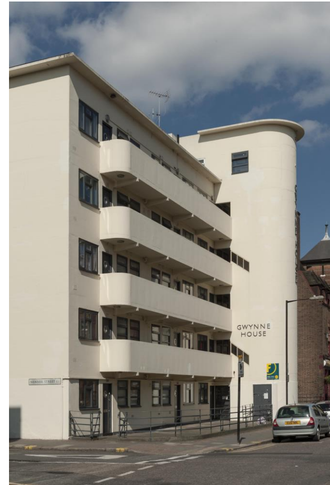
View of Gwynne House from the south-west.
