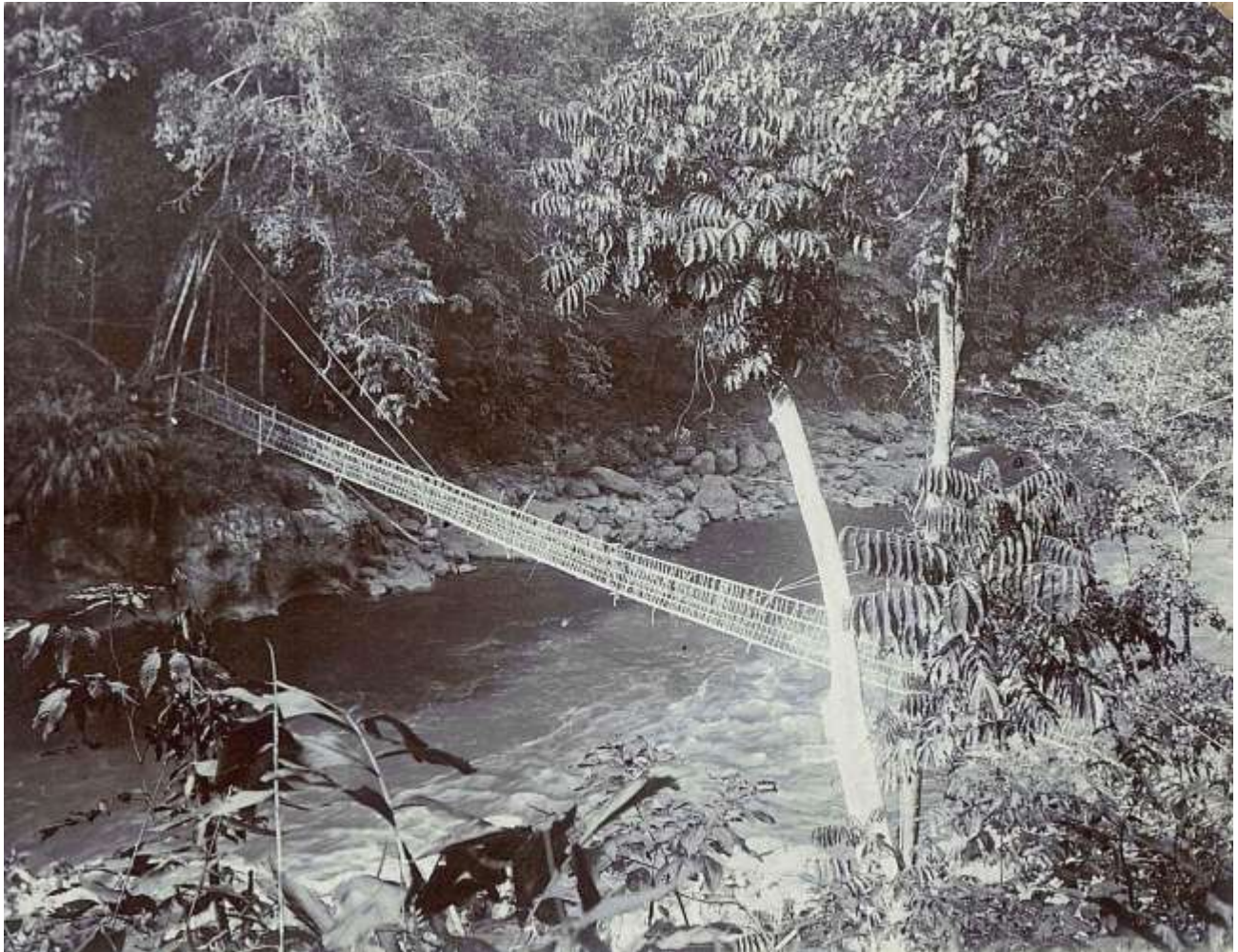
Figure 2. Rattan pedestrian suspension bridge in the Malaysian rain forest before the First World War. From the archives of Fred Aldous Ltd, Manchester who have traded in rattan since 1860.
