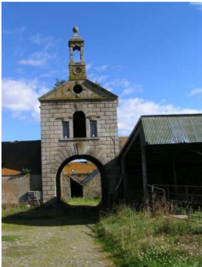
Figure 5. Entrance to the Mains of Carnousie, built 1797. Image courtesy of Alistair Mutch.
