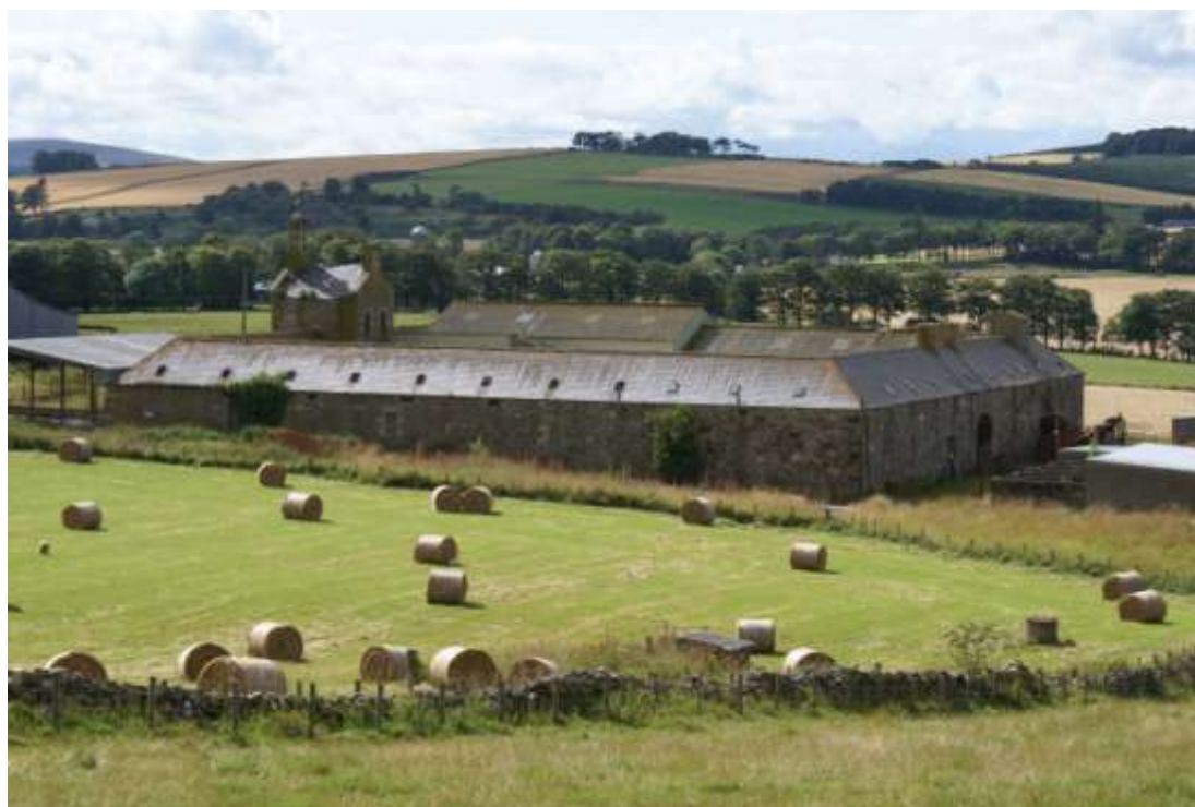
Figure 8. Mains of Carnousie steading. Note gate house in left corner, leading to arches mentioned above. Image courtesy of Alistair Mutch.
