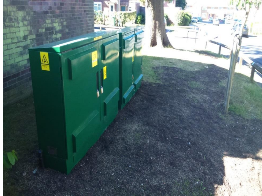
Erect ESMU, connect and commission
