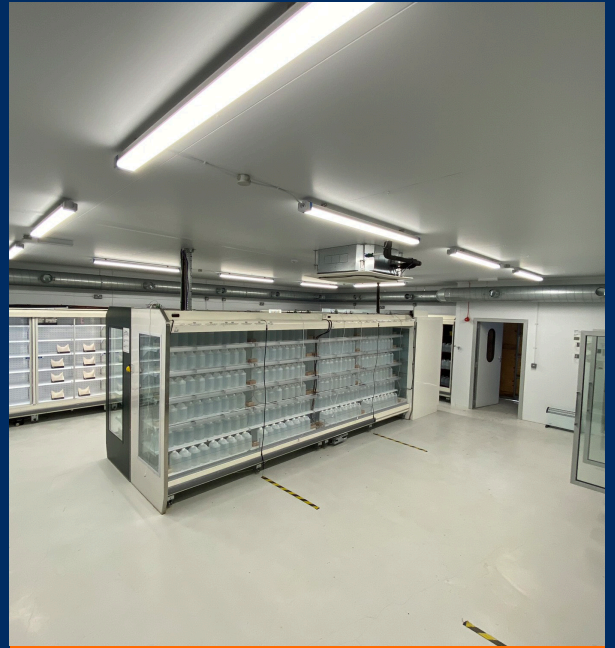
Refrigeration Research Centre
