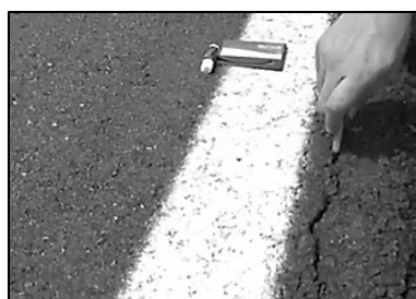
a. Visual survey (cracking)
