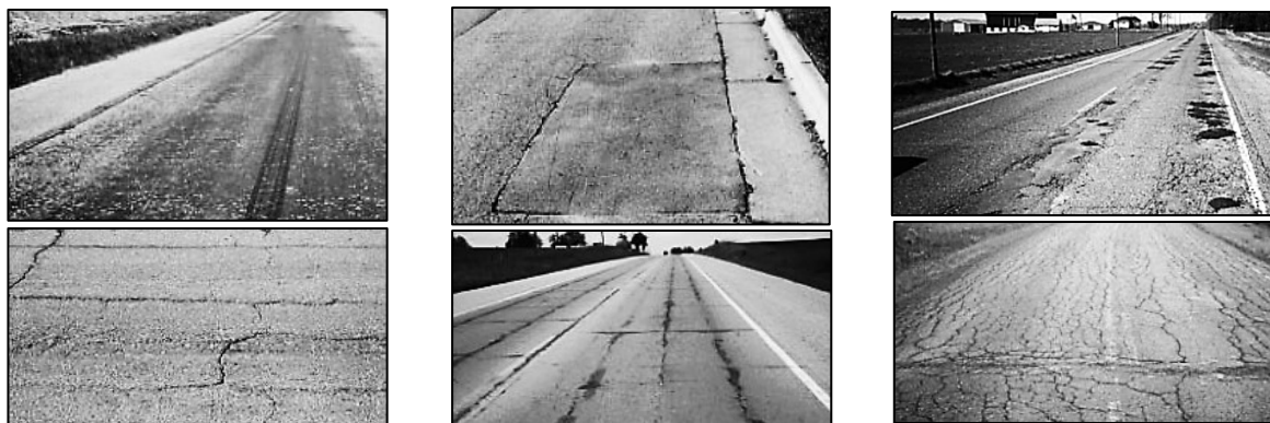
d. Rating 5: Fair / extensive bleeding, medium ravelling, cracking of medium severity (but still in good structural condition)
