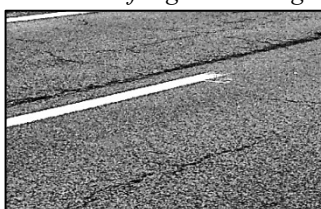
h. Cracks next to longitudinal joint
