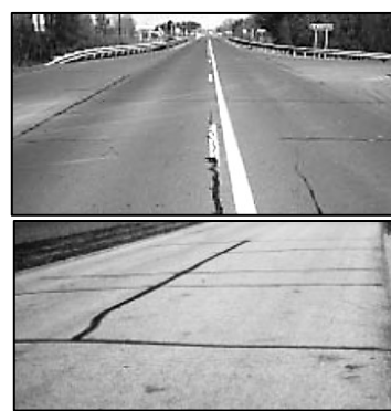
c. Rating 7&6: Good / signs of ageing, sealed cracks of low to medium severity, slight ravelling
