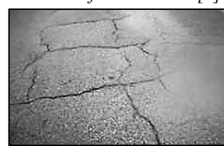
f. Block cracking
