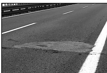
a. Localised pothole patch
