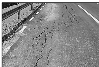
k. Multiple cracks and mud pumping
