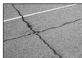
c. Joint reflection crack [5]
