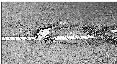
c. Severe slippage caused by debonding [38]
