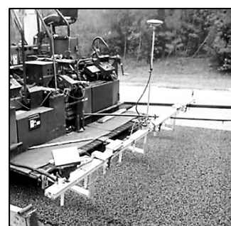
c. IRT measurement of HMA overlay [32]
