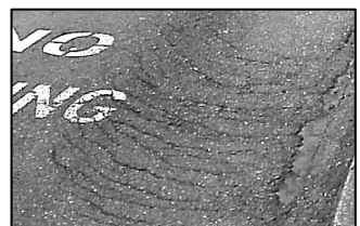
g. Slippage cracking
