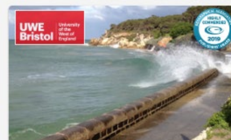
Hard engineering approaches to coastal management Coasts - Knowledge Booster
