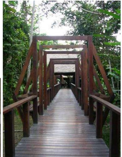
• constructed from local materials (selectively felled timber, palm fronds)
