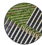
Vertical monocrystalline solar panels and solar water heating are positioned between timber slats, on 45° south facing roofs. To the north are extensive green roofs helping water runoff and biodiversity.
