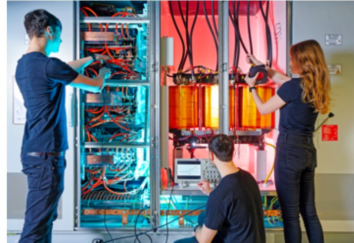
5,0 MVA, 1.000 Hz Transformer 675 kg (0,14 kg/kVA)
